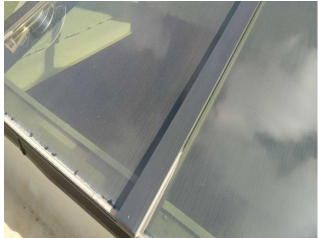
After all sections were water tested, we water tested each of the skylight systems
