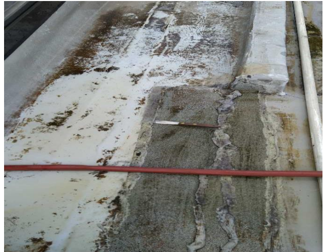
Active leak location #1
