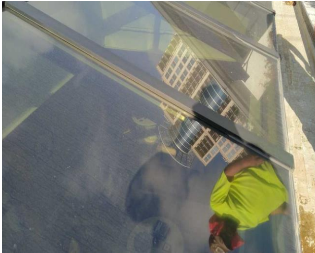
After all sections were water tested, we water tested each of the skylight systems
