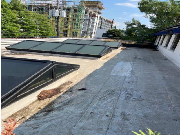
General view of the existing roof conditions
