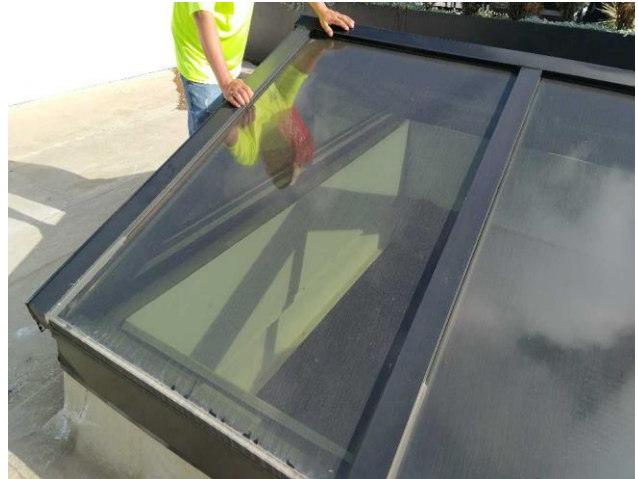
Active leak location #2. After all sections were water tested, we water tested each of the skylight systems. We found missing sealants at various locations of the skylights
