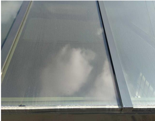
After all sections were water tested, we water tested each of the skylight systems
