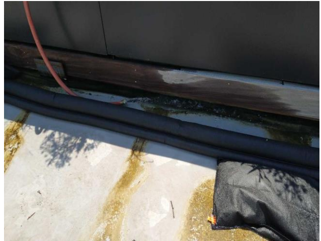
At each section, we dammed off the areas to isolate the standing water to each of the sections
