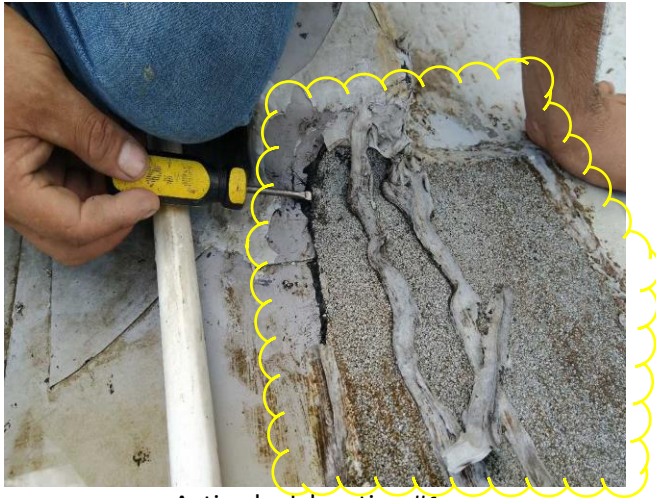
Active leak location #1
