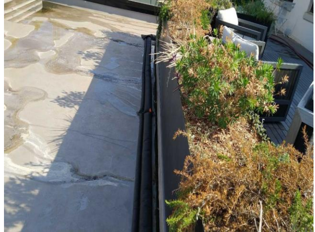
Performed water testing at planter #1-2 section
