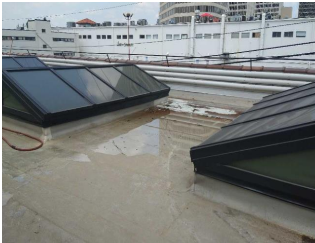
Each section that was water tested, we had a minimum of 2" of standing water on the roof over a period of time
