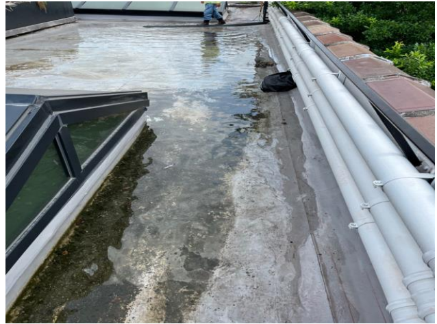
Each section that was water tested, we had a minimum of 2" of standing water on the roof over a period of time
