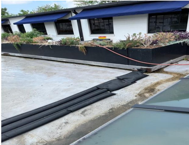
Water testing the planters
