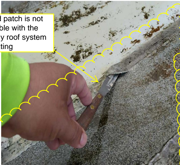
Active leak location #1
