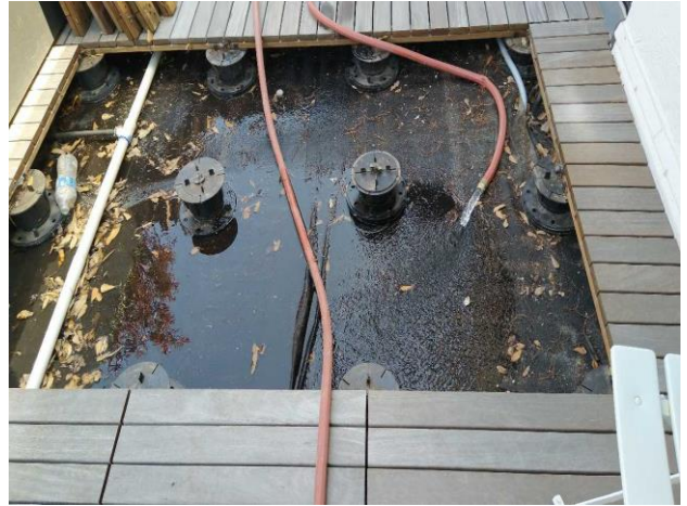
Performed water testing at section 6, 7, 8, 9 and 10 at only the wood plank locations where it butts up to the planters
